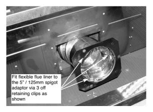
Re-fit the 5" / 125mm flue spigot adaptor into the top of the combustion chamber, and secure with the four M4 screws as shown below in Fig. 15.
