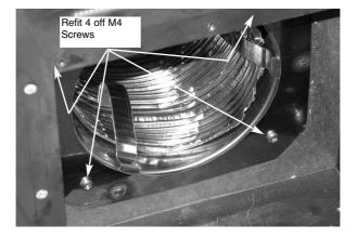
Re-fit the draught diverter and secure with the five off M4 screws as shown below in Fig. 16
